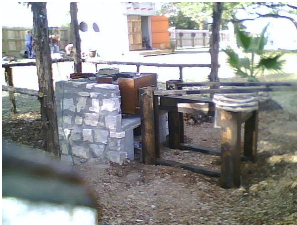
Figure 10 – The Bellows installed
