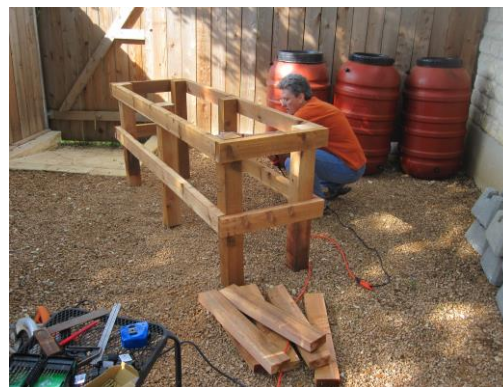
Figure 2 Securing screws on frame
